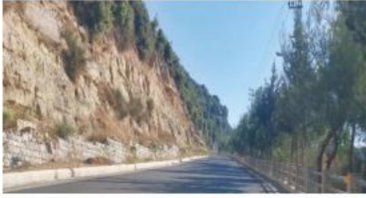
Deteriorated top of wall due to rock falling
