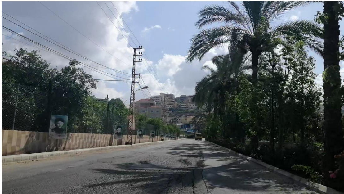
Figure 3-15: Road L3-SO-RD08 (Abbasiyeh village)
