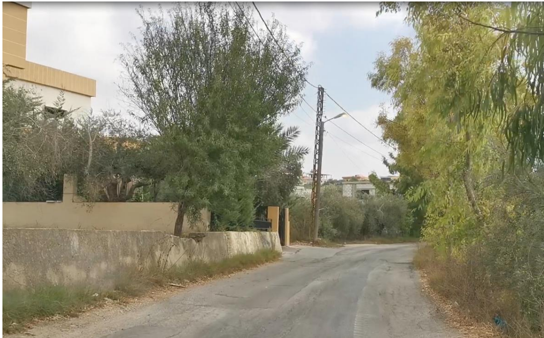
Figure 3-13: Road L3-SO-RD06 (Chhour village)
