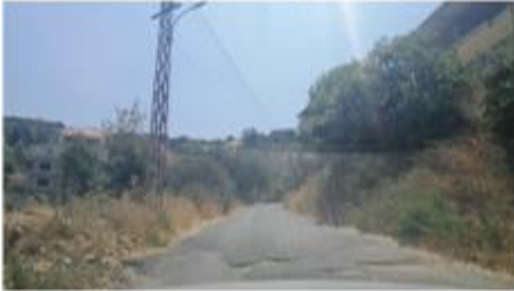
Hasbaiya Road 3 – Sta 0+850
