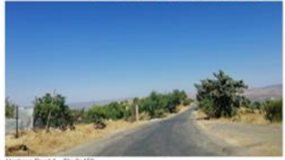
Hasbaiya Road 1 – Sta 0+150
