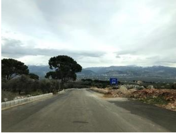
Road 1a-Btorram (34°20'40.2"N 35°48'11.2"E)
