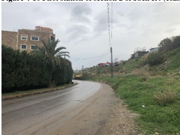
Figure 4-10 First station of section 2 of Jbeil R4 (coastal section of the road station 0+000, Baachta)
