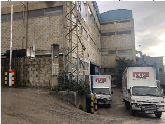
Figure 4-7 Industrial area bordering the road, Section 1 (stations 0+000 & 3+000-Jbeil R4)
