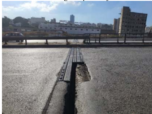
Photo 2 Levelling of surface below the expansion joint
