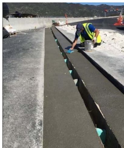
Photo 2 Levelling of surface below the expansion joint
