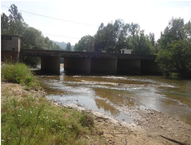
Hydraulic Structure Entrance
