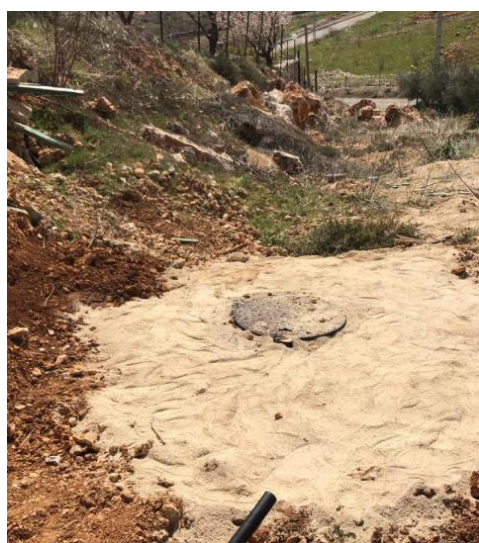
Figure 10: HZ-KA to be adequately backfilled and stone retaining wall to be rebuilt
