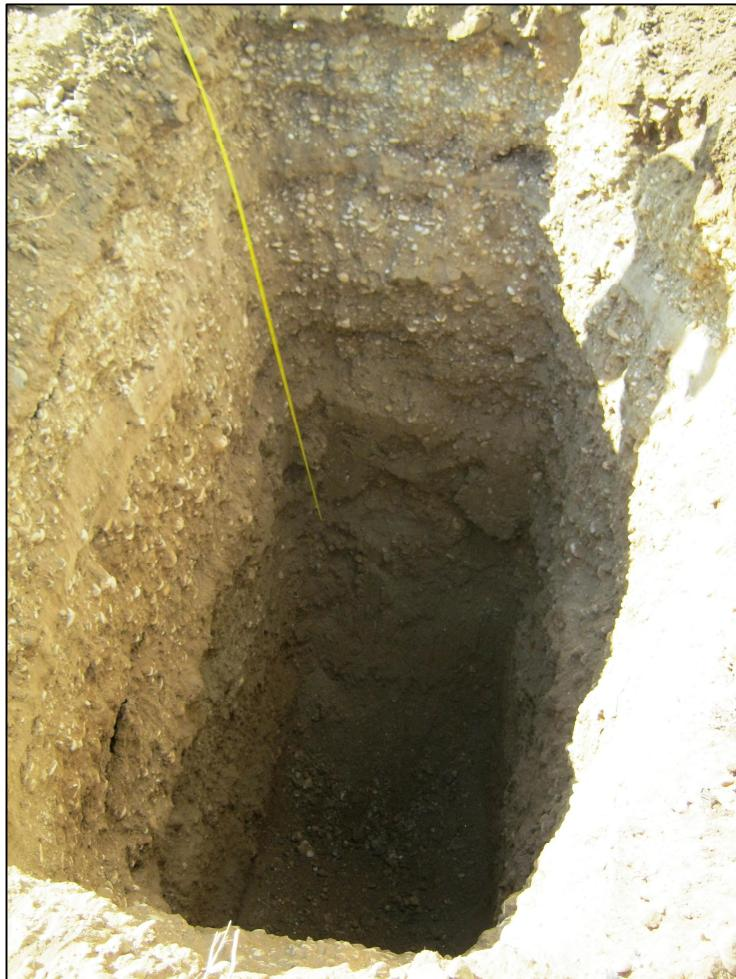
Figure 3: NTP11, Sand/Gravel material source of S-4
