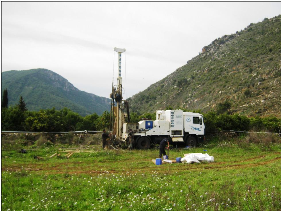
Figure 5: Truck mounted drill rig used in coring (BHVR3).
