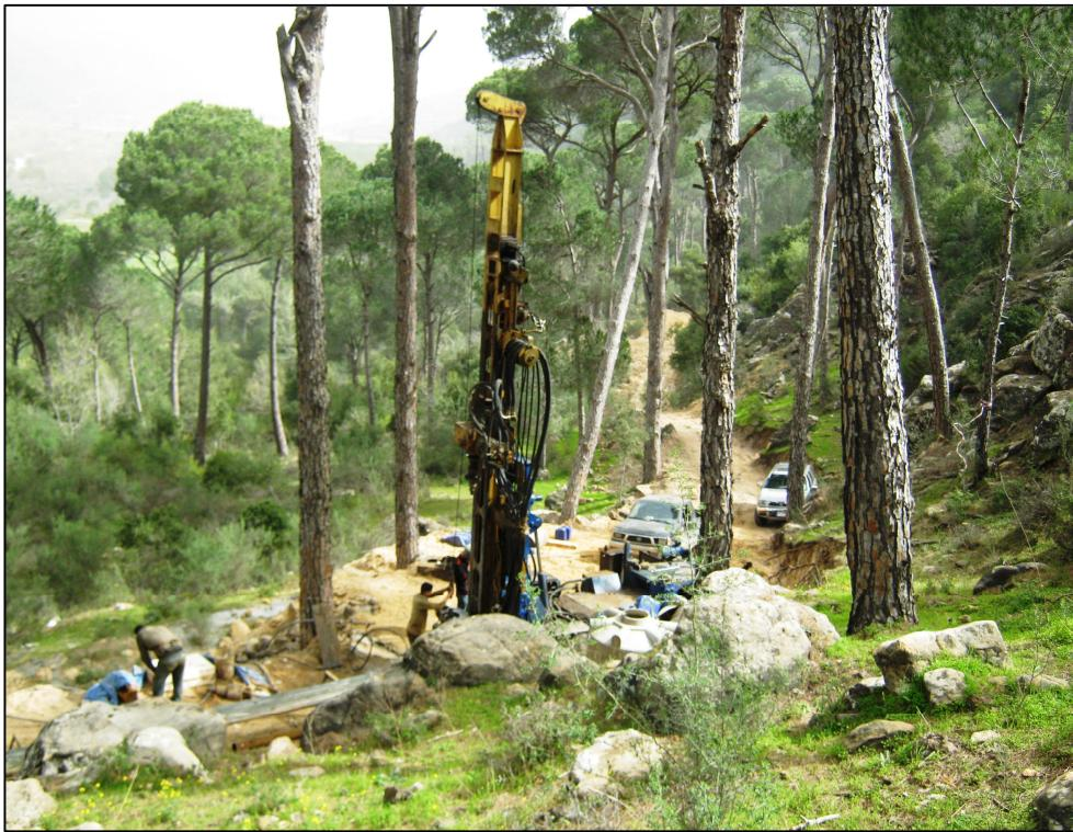
Figure 3: Crawler mounted drill rig used in coring (BHLA2).
