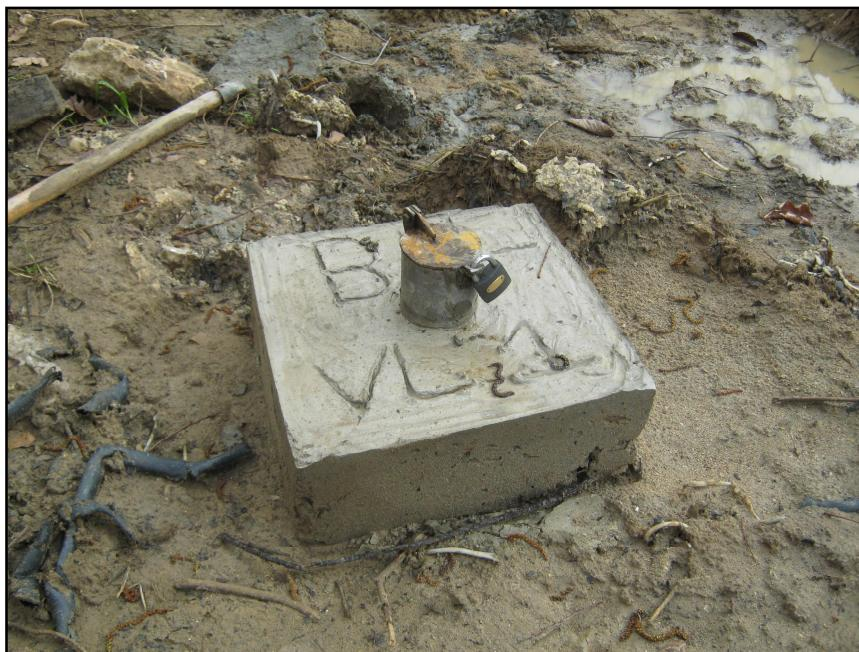
Figure 15: Concrete heading and steel pipe protection
