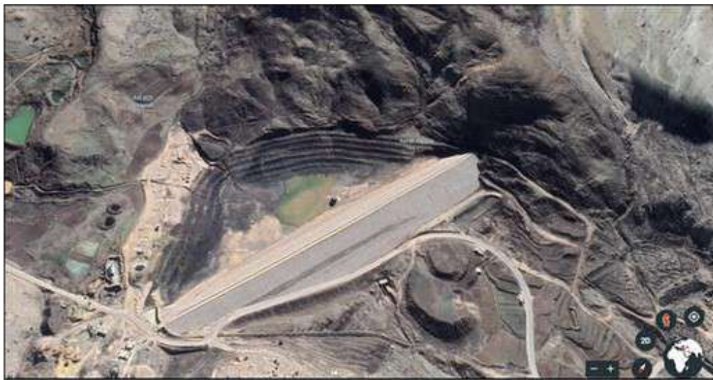
Figure 1: Aerial View of the Existing Brissa Dam
